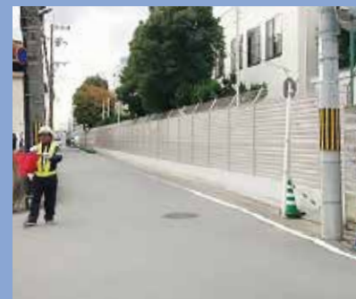
After the safety measure (Head Office)
