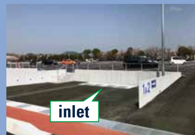
Elevated parking lot (Inuyama)
